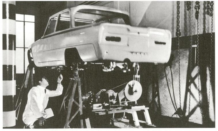
THE PAVEMENT TEST - The frame is firmly secured at three points: at the fourth point a type of piston repeatedly pushes the body up and down. This has the same effect as if one wheel of the car
